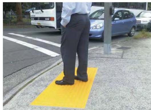
The intended application for this mode is without the optional vehicle loop and is for “passive pedestrian detection” at signalised pedestrian crossings.
