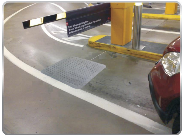
New SMR-900 utilising existing Lead Wire slot
